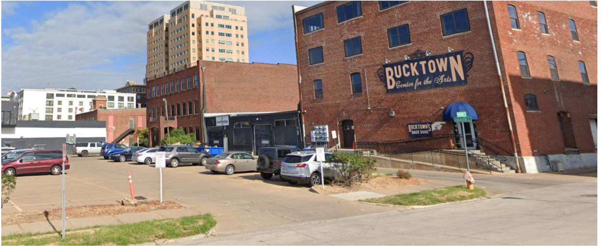
East Elevation from Pershing
