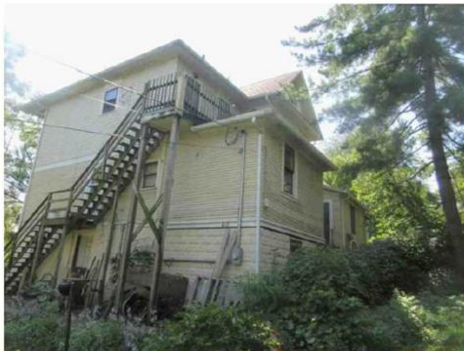
North & West exterior
