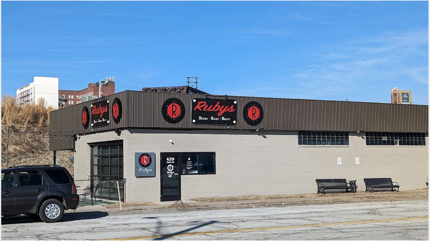
Rubys Exterior South and West Elevations Before PXL_20230226_154432485.MP.jpg
