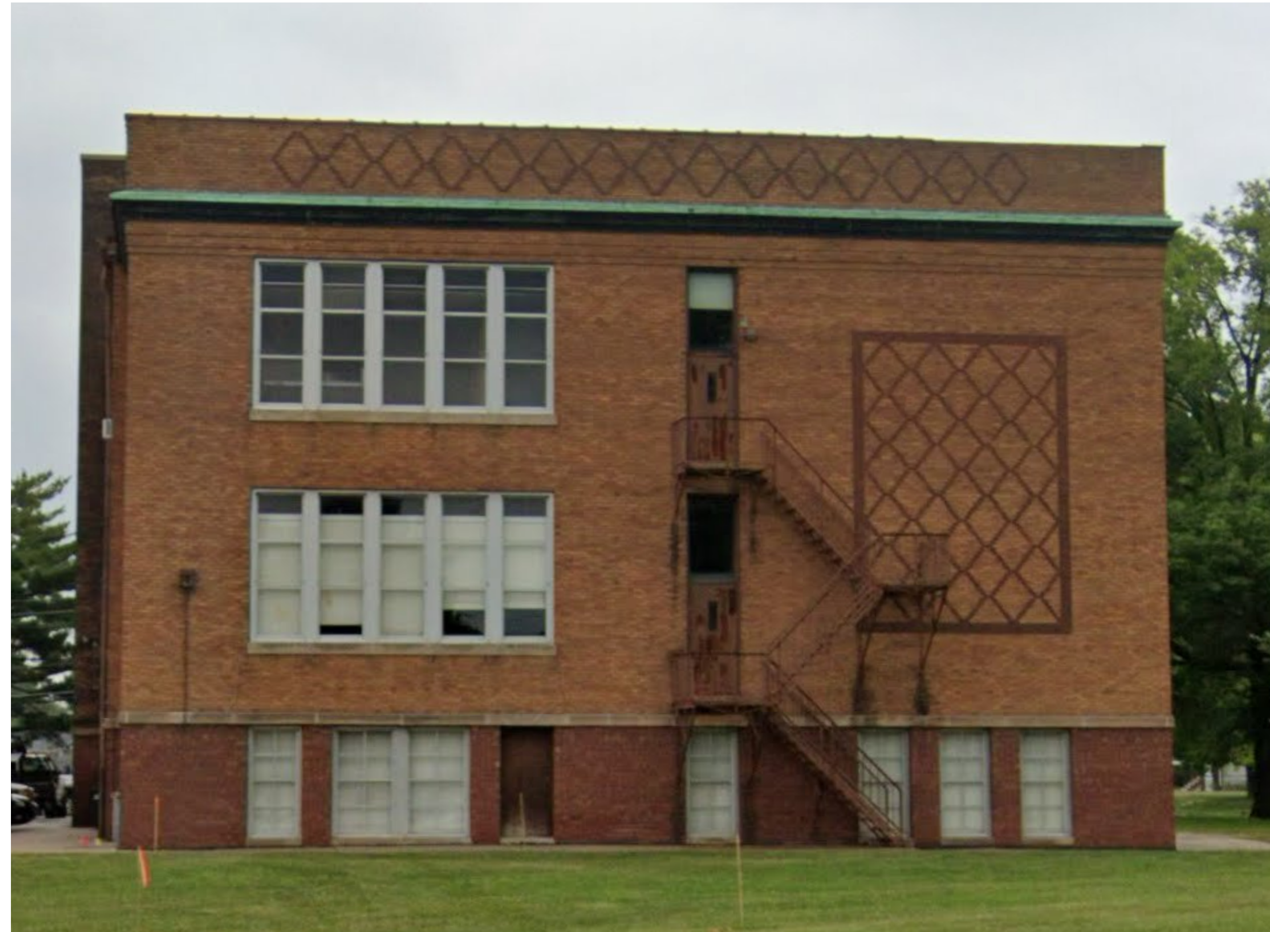
Elevator Shaft Location A
