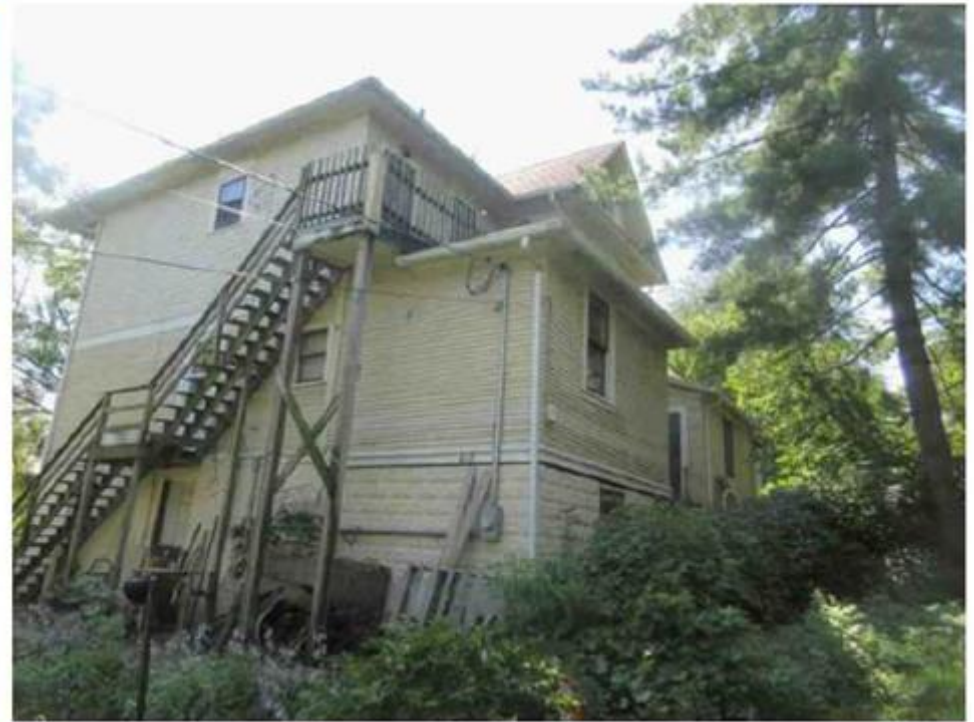
North & West exterior
