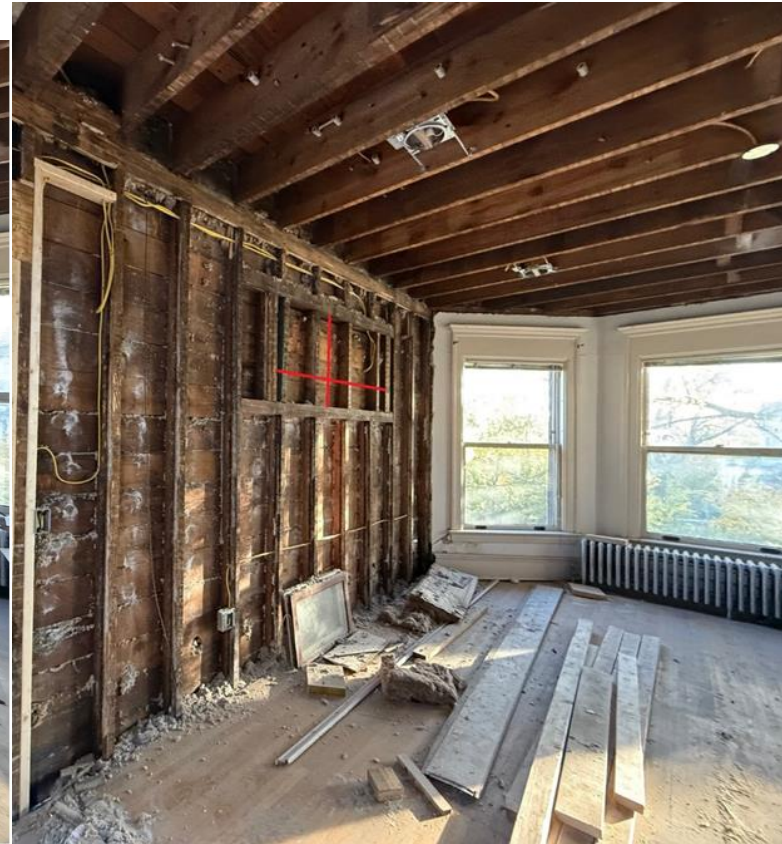
NORTH INTERIOR WALL DINING ROOM HIDDEN ORIGINAL EXISTING WINDOW ROUGH-IN FRAMING
