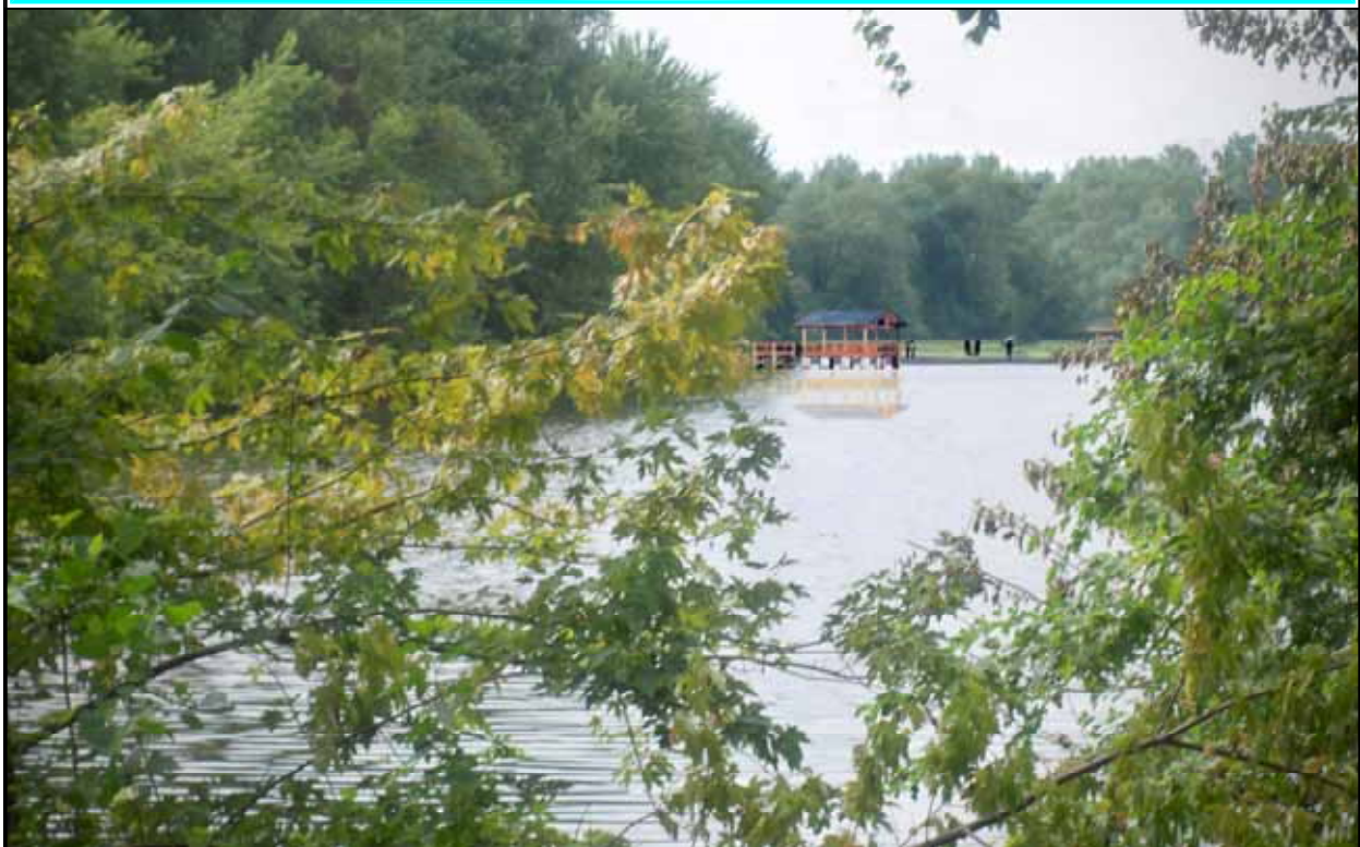
AREA 7a - LAGOON PAVILION (AFTER)
