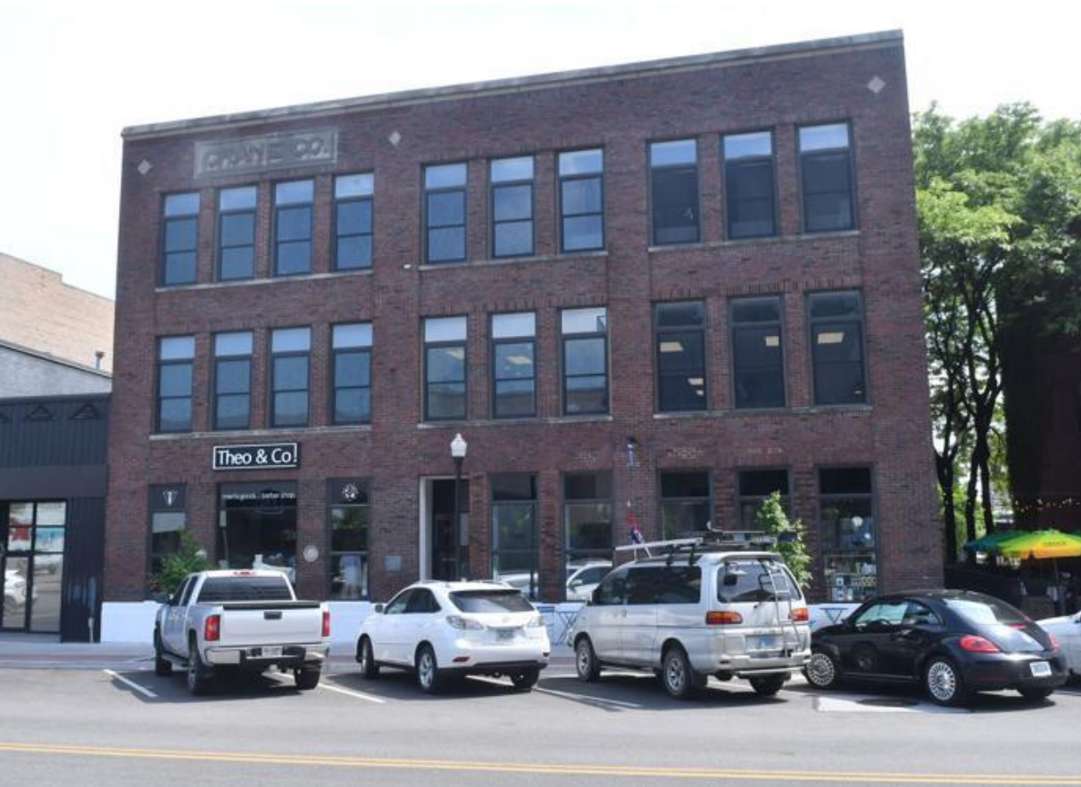
North Elevation East 2 nd Street
