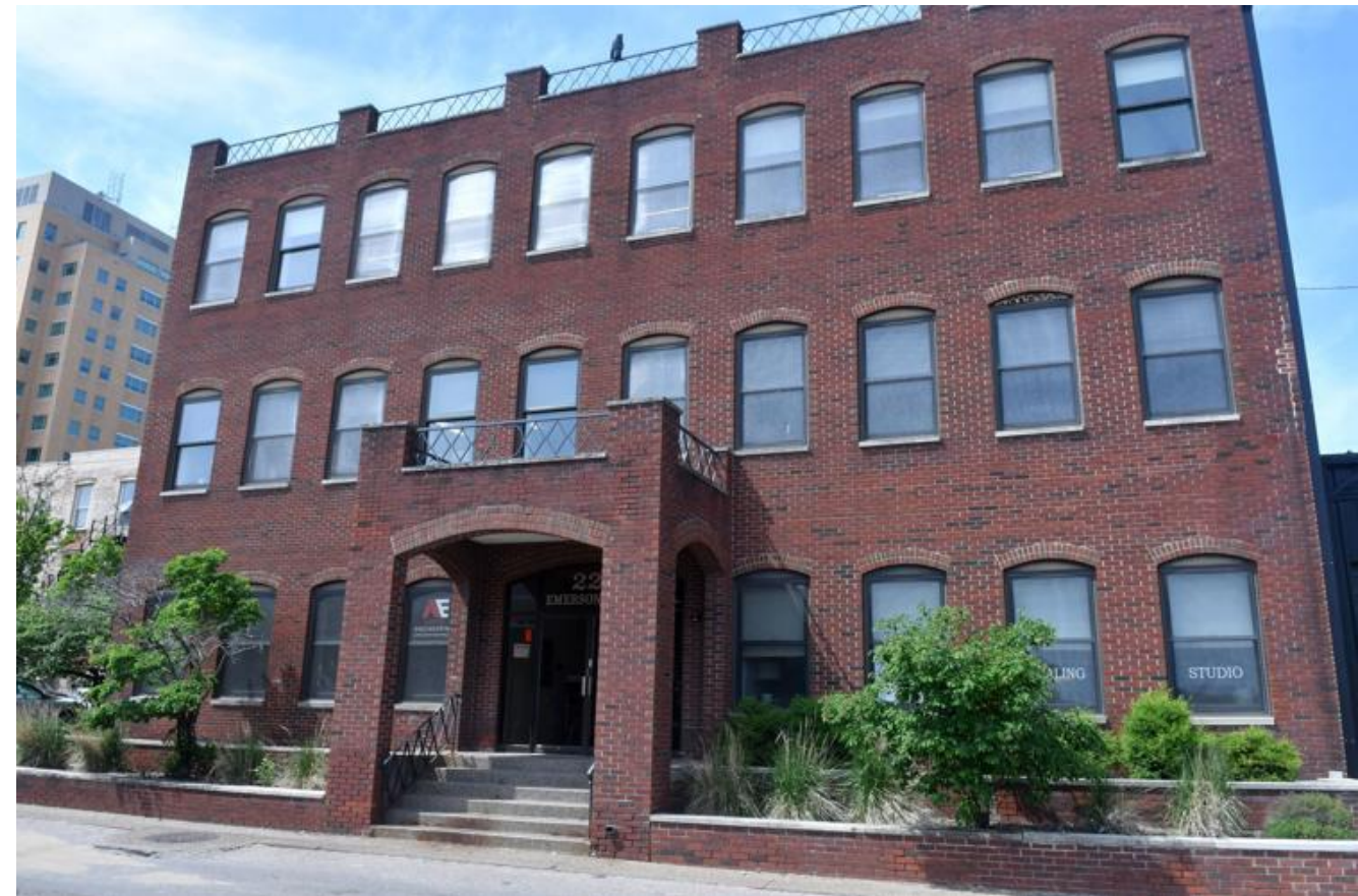
South Elevation - Emerson Place Entrance to Bray Architects Office
