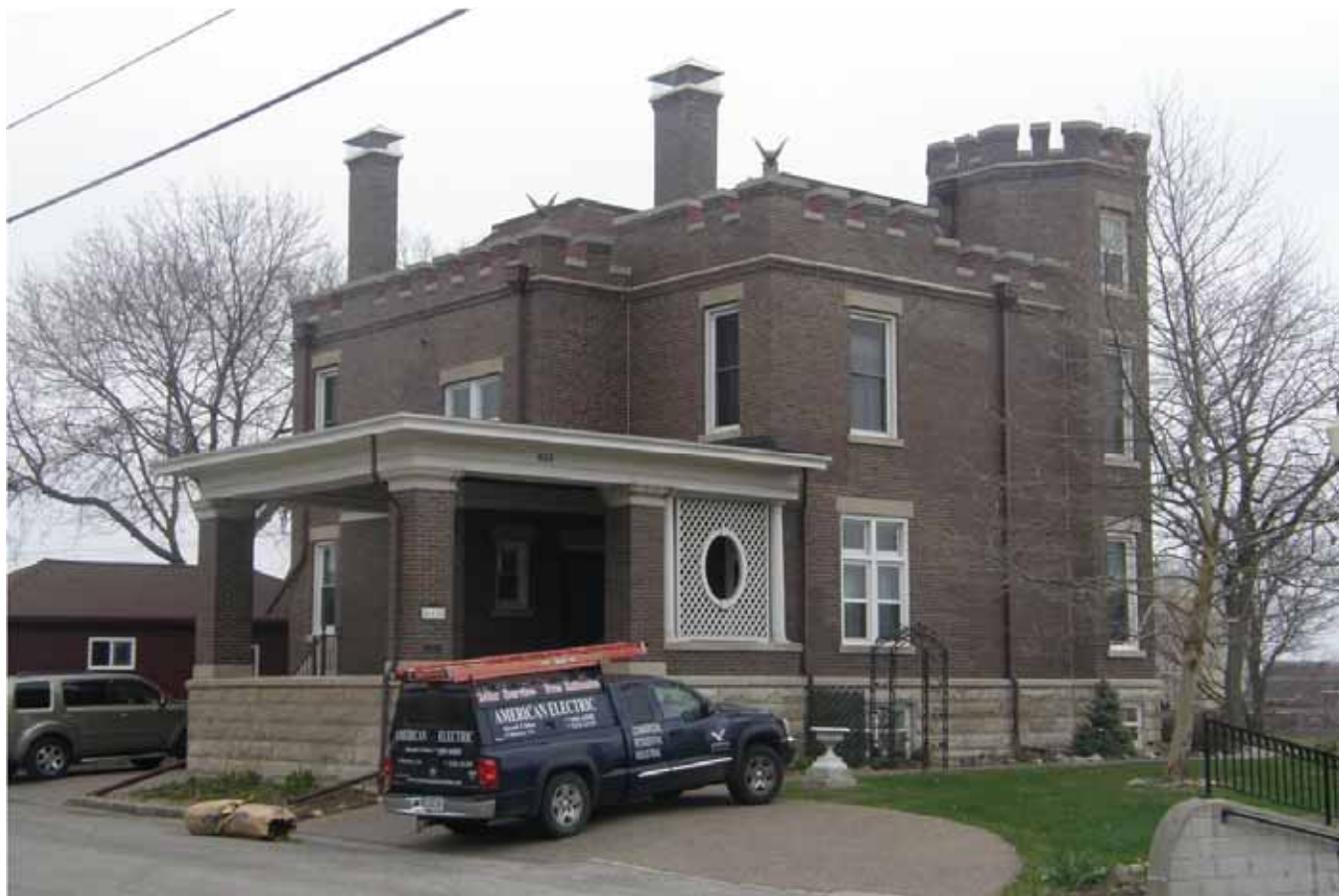
Photograph 82-02494-003 - House, looking southeast (April 2015)
