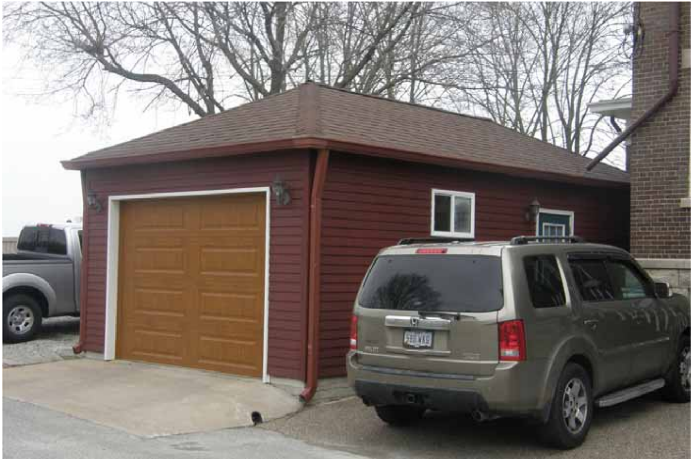
Photograph 82-02494-004 - Outbuilding, looking southeast (April 2015)
