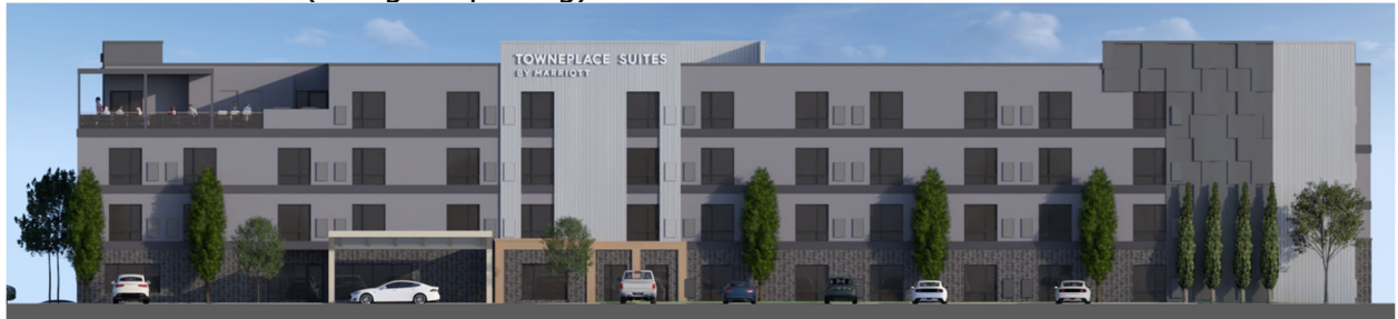
Hotel East Elevation (facing the parking)
