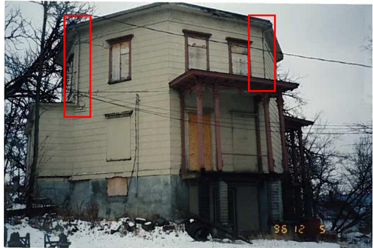
1996 Photo of the Octagon House Evidence of Downspouts
