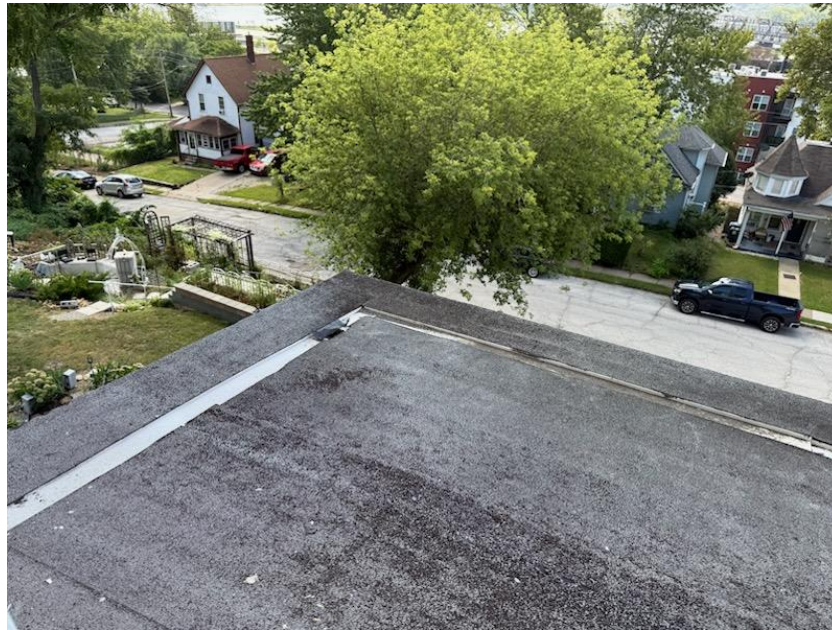
South Porch Material: Rubber Membrane
