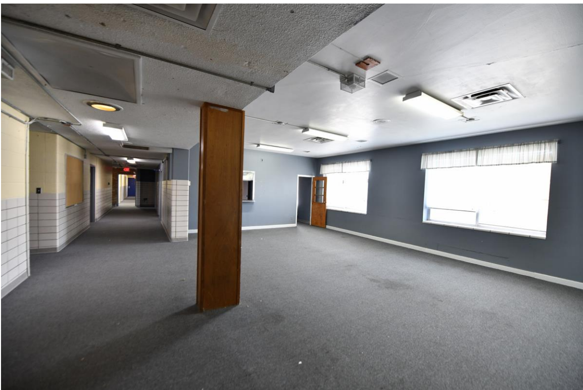
Children's Cottage | Interior | Typical Interior
