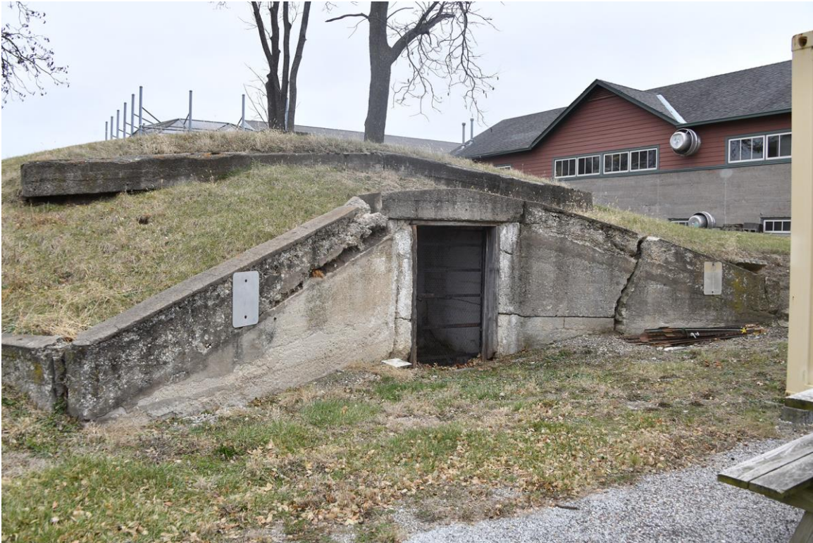
Root Cellar | View East
