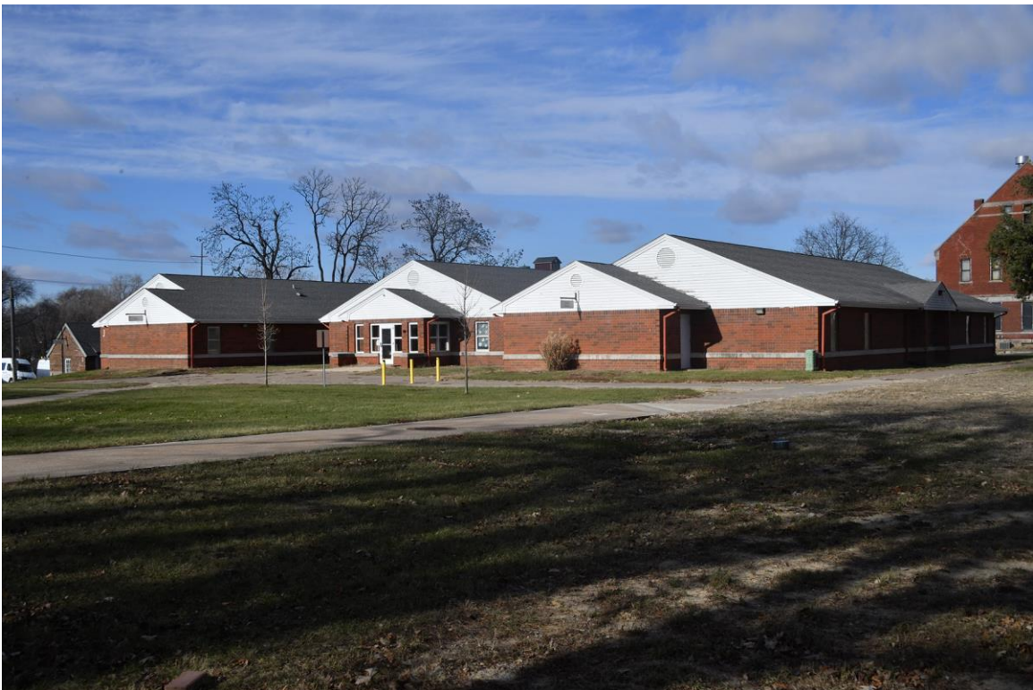
Leslie Building | View Northwest
