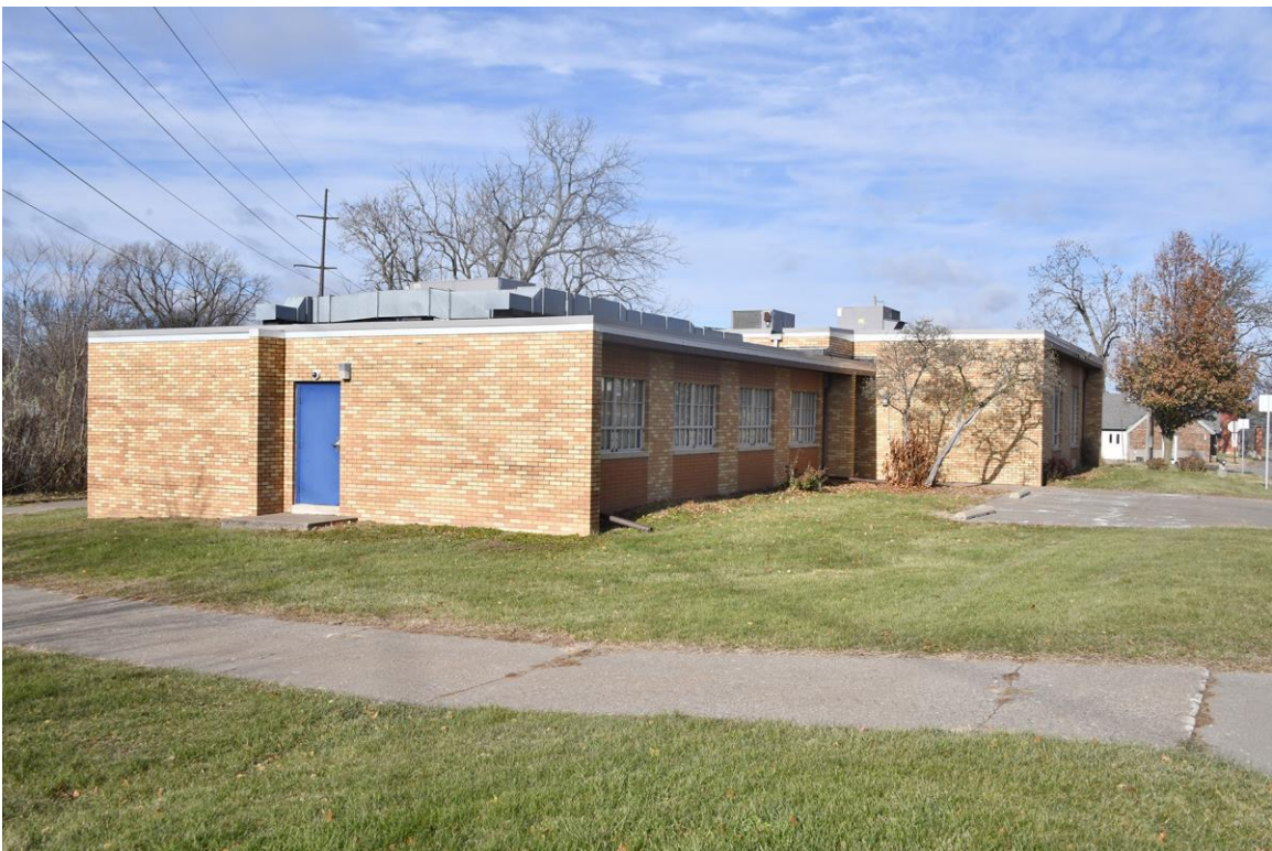
Children's Cottage | Southeast Corner | View Northwest
