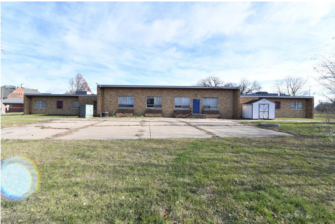
Children's Cottage | Rear West Elevation | View East
