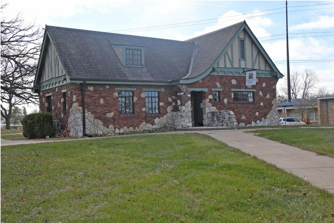
Pre-School/Porter Building | View Northwest
