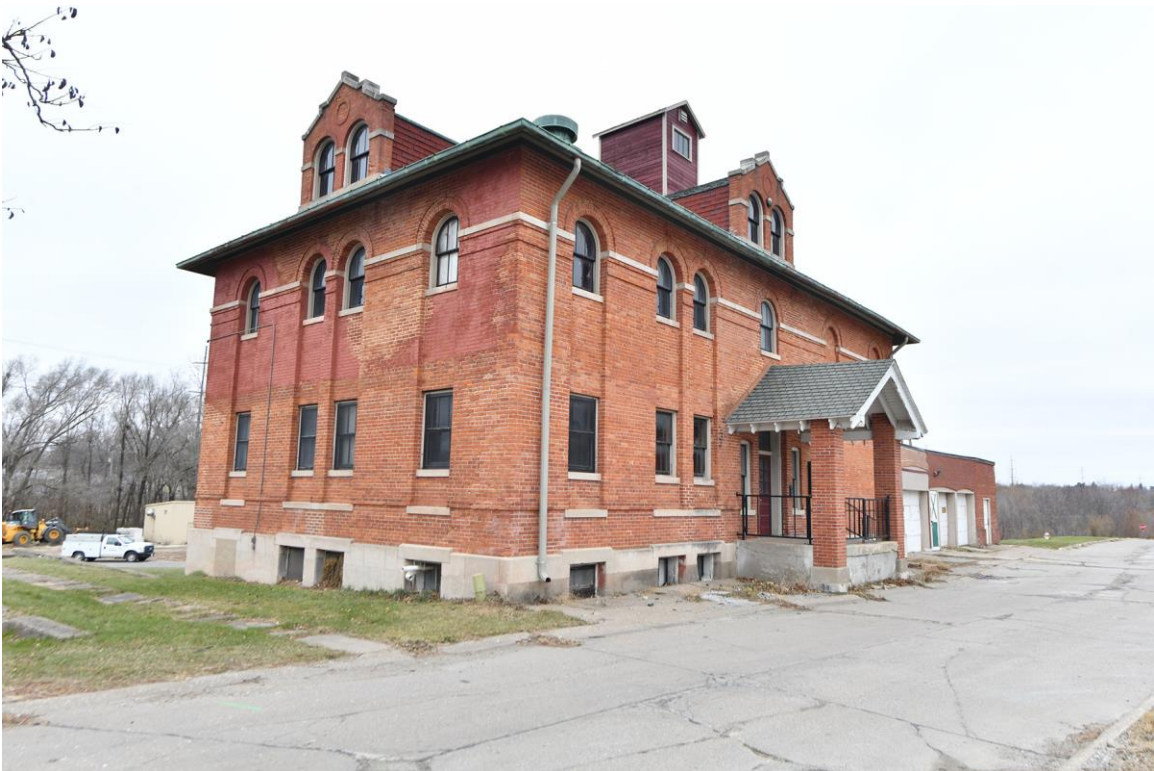
Ice House-Storage Building | View Northwest
