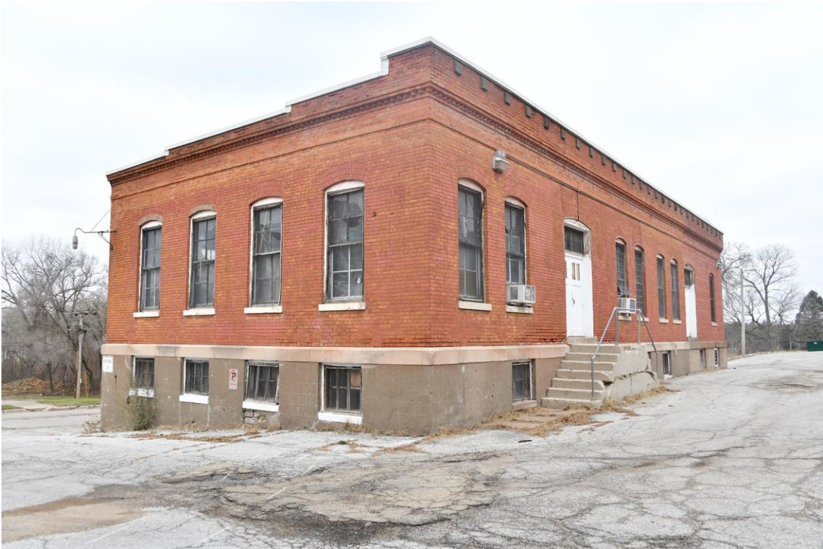
Boy's Manual Training Building & Work Shop/Carpentry Shop-Blacksmith Shop/ Maintenance Building | View Northwest
