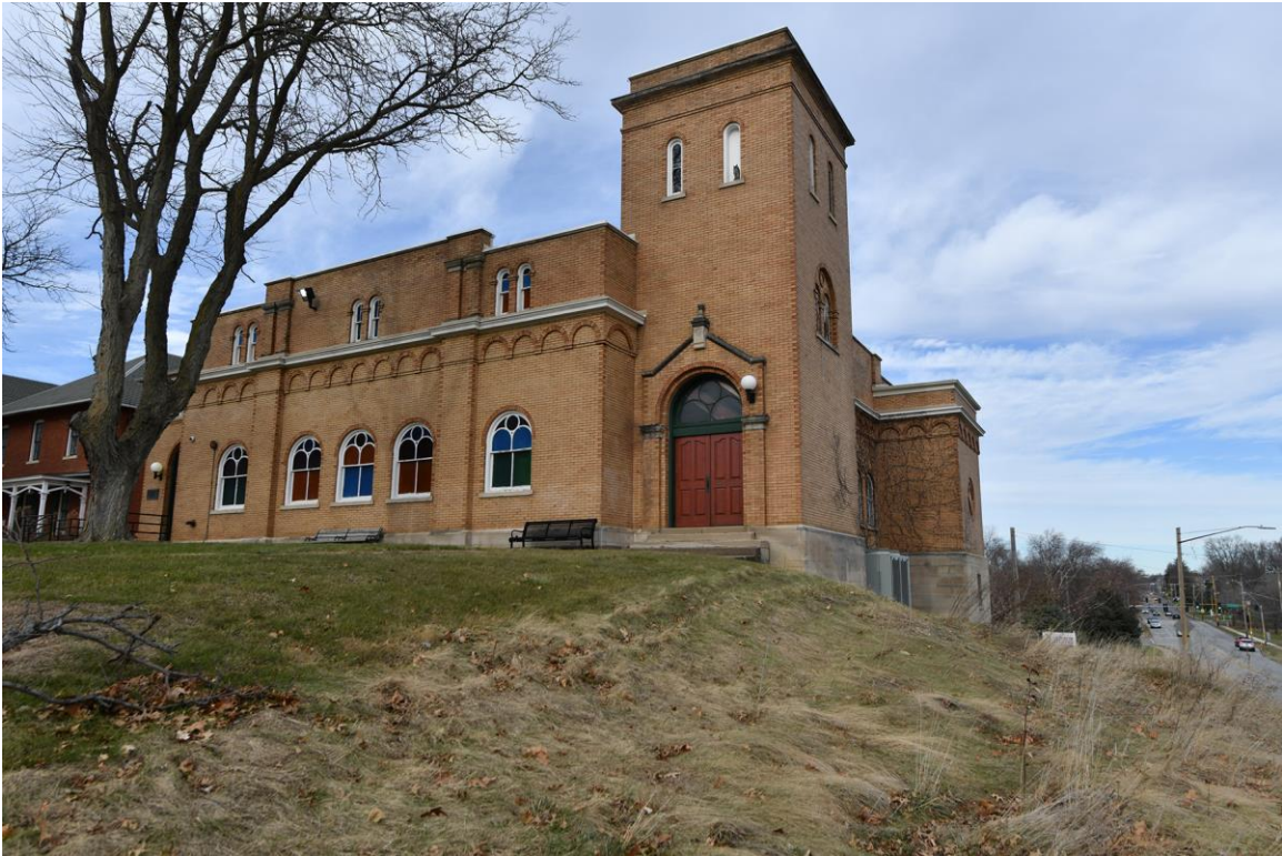
Chapel | View Northwest
