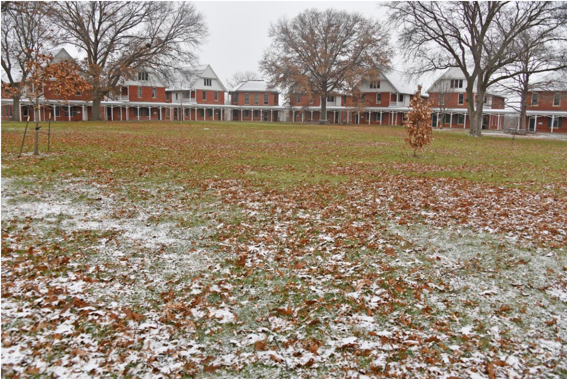
Rear of Boys' Cottages | View Northwest
