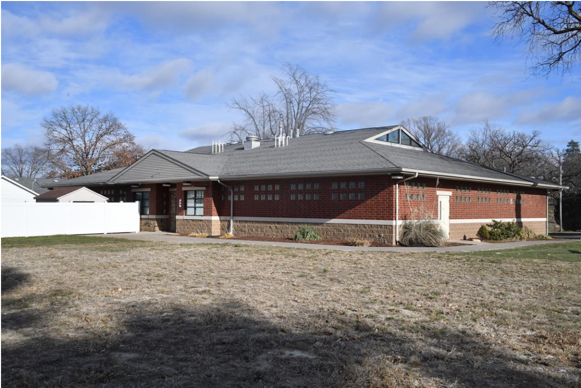
Boyd Building/Shelton Building | View Northeast
