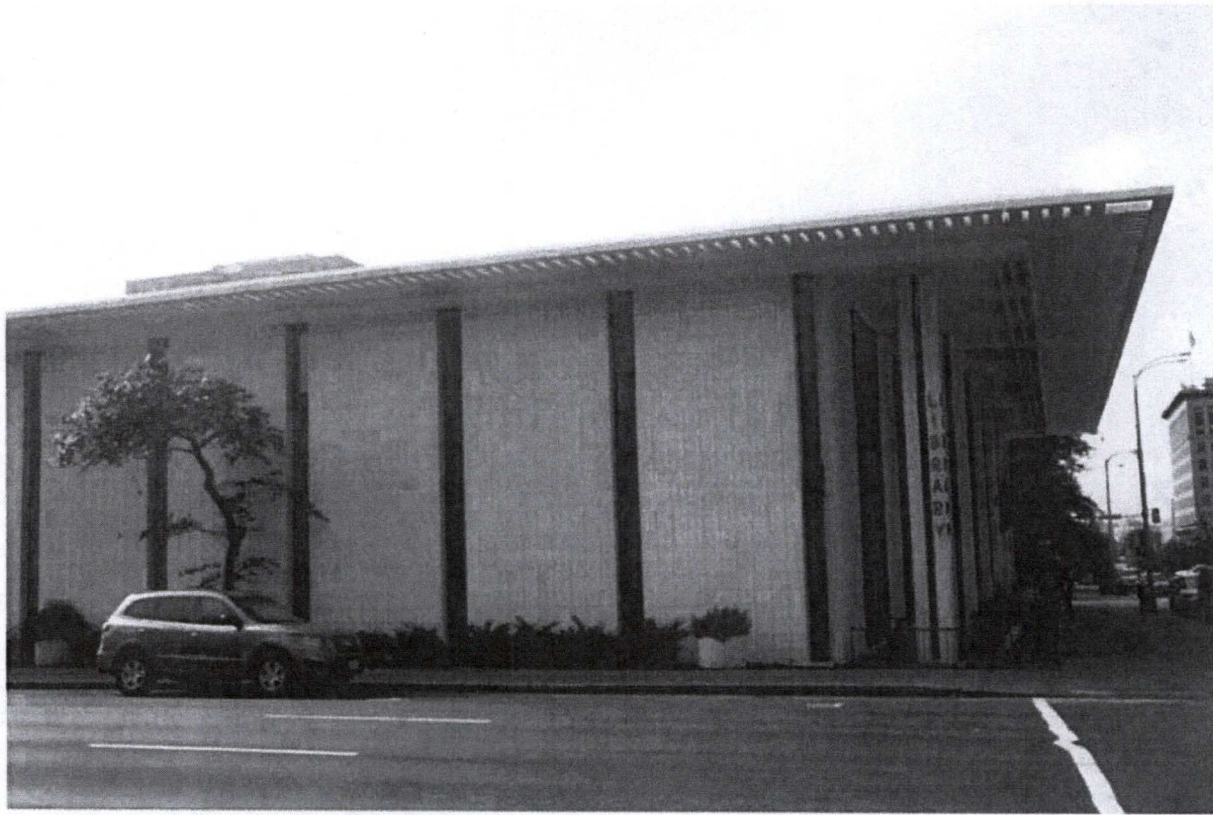
View from the north west corner. This image shows the slitted overhang that Stone used in many of his designs. (Sept 2018)
