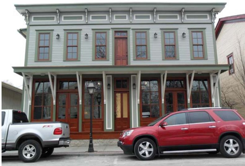
The rehabilitation of this building is expected to be completed in 2013.
