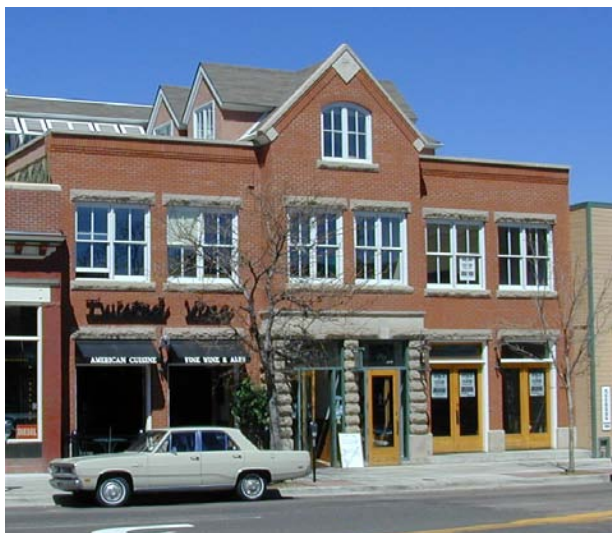
Incorporate traditional building components such as a base, middle and cap into the design of a new building (Boulder, CO).
