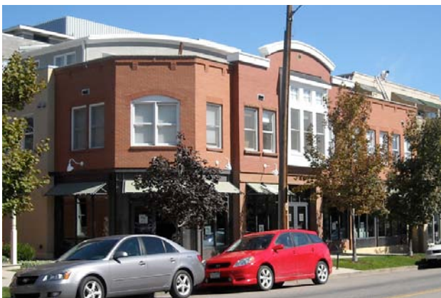
Use high quality, durable building materials, such as masonry brick for commercial buildings (Boulder, CO).
