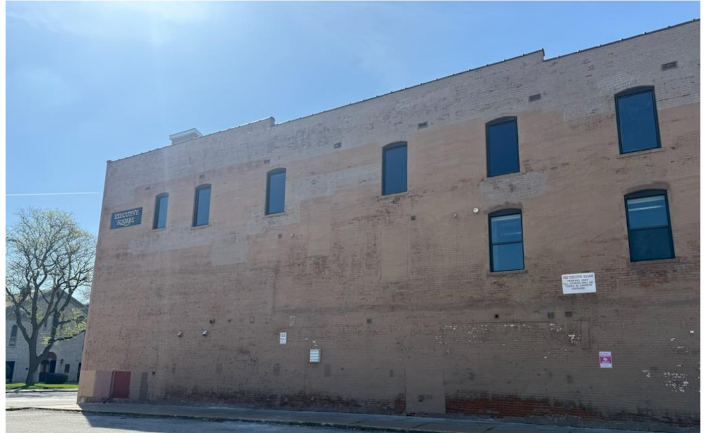
Repaint North Facade
