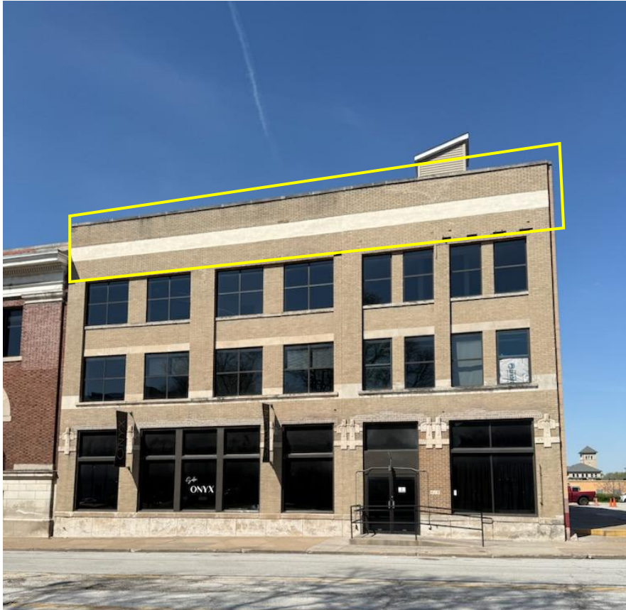
Reconstruct East Parapet Wall
