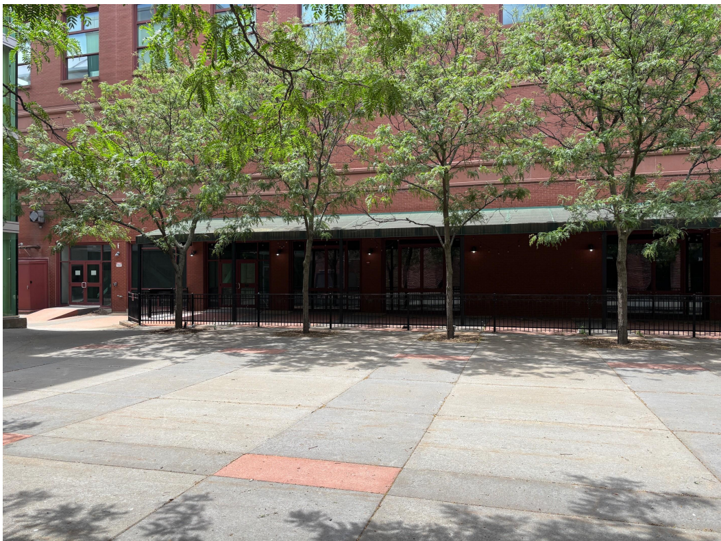
Existing east facade; standing in courtyard looking west
