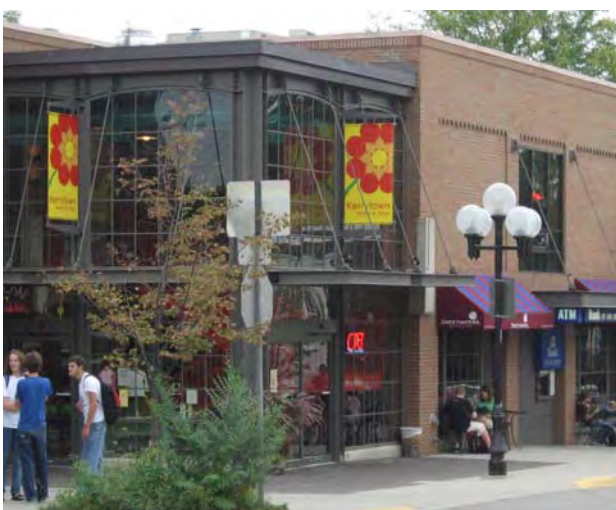
A contemporary addition to the south of the historic building, would be an appropriate design approach. Materials should be of high quality (Ann Arbor, MI).
