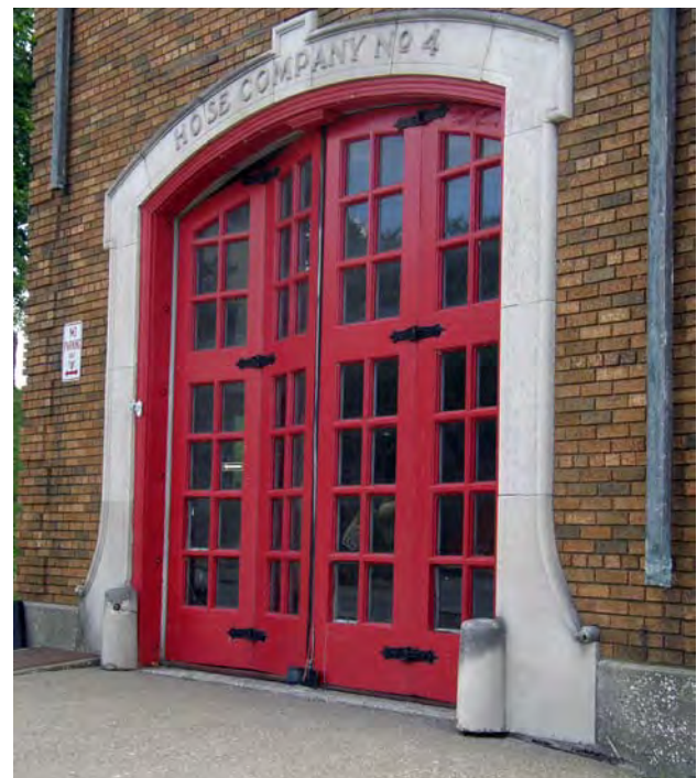
Hose Station No. 4 is a distinctive historic landmark that anchors the eastern edge of the Village core.
