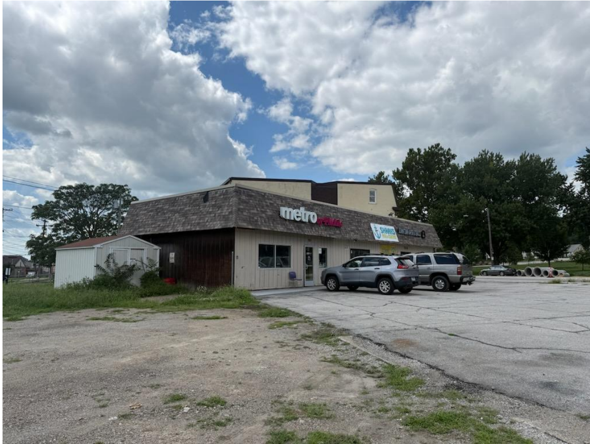
Southeast Elevation – Facing Gaines Street
